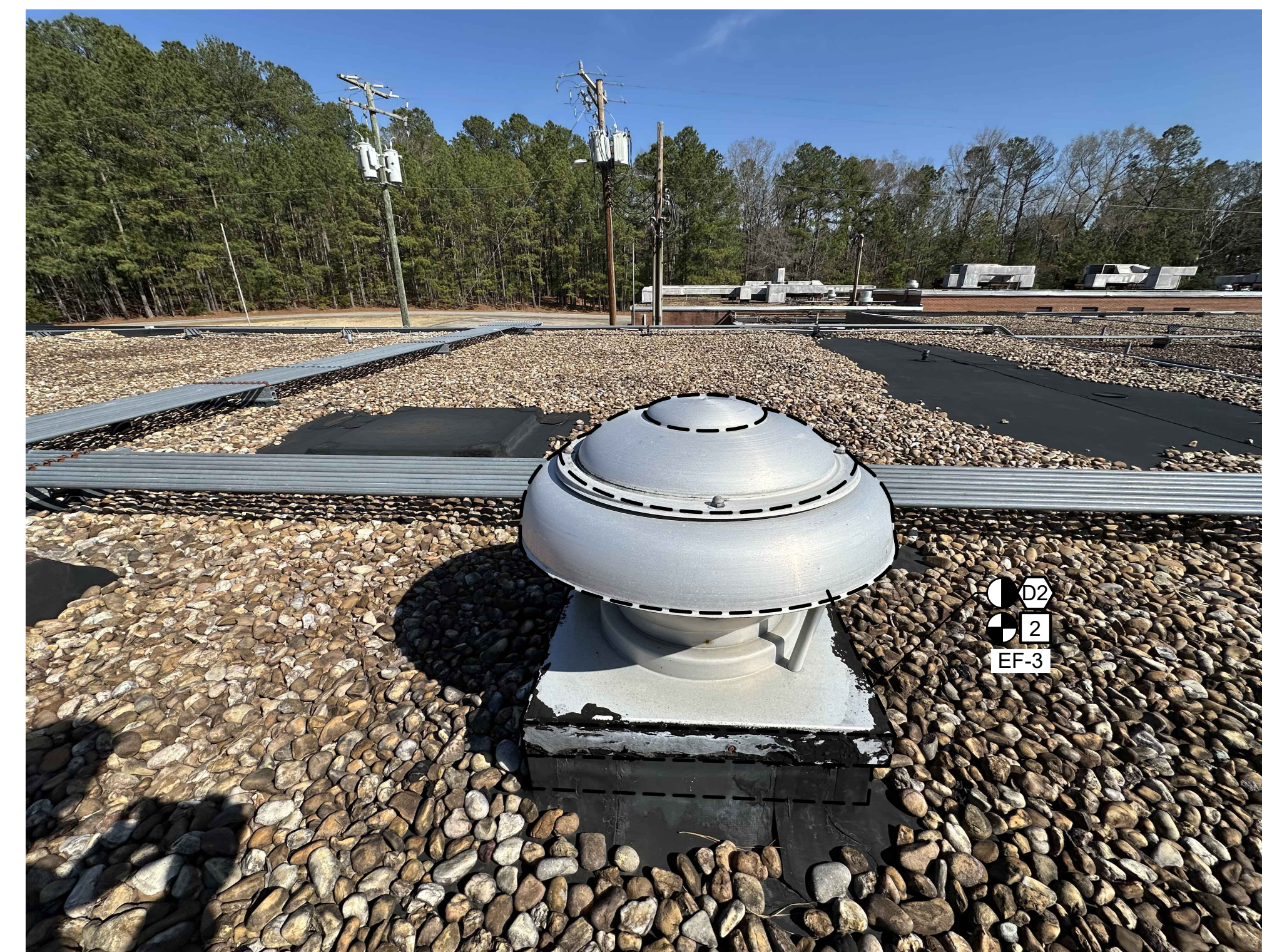
P3 TYPICAL EXHAUST FAN REPLACEMENT PHOTO M1.1 NOT TO SCALE
